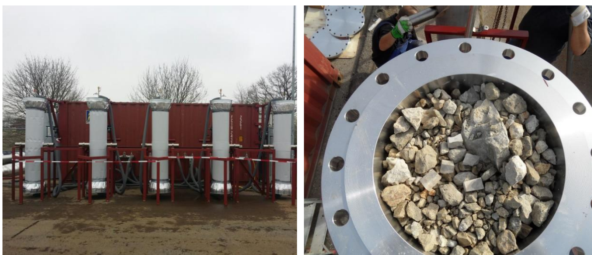
Fig. 2 (a) Bypass system in Kirschweidach and (b) Reaction columns while being set up
